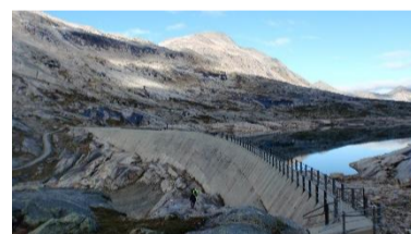
Dam Reinokvatn, Statkraft/Photo: Thomas Konow, Dr.techn.Olav Olsen
