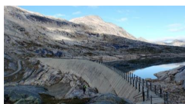
Dam Reinoksvatn, Statkraft/Foto: Thomas Kanow, Dr.techn.Olav Olsen
